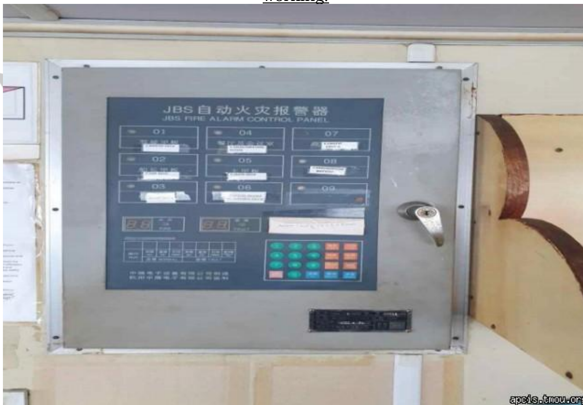
Picture of other detainable deficiency: Fire detection alarm system not working.
